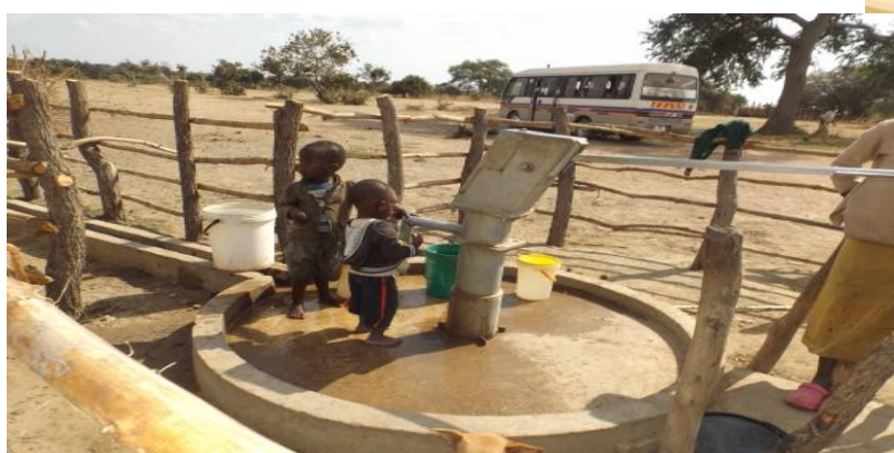
Left - Borehole was poorly constructed fitted with a manual handle instead of a solar powered handle connected to a tank. And Right Mr Joel Hang'omba, a small scale farmer responding to the PETS Committee Report findings.
